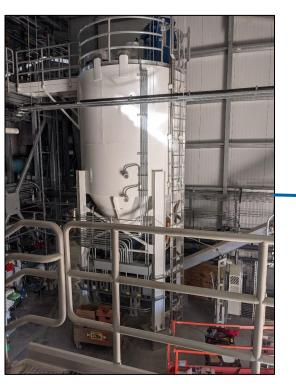
Large Capacity Systems Silo +Feed Auger
