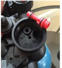
Be sure the proper **Drain Line Flow Control Button** (DLFC) is installed in the control valve and that the button is installed in the correct orientation, the rounded bevel edge is facing the water flow from the control valve to the drain.
