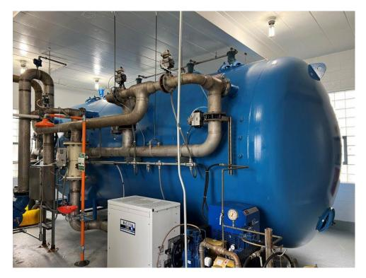
Figure 9: Well 8 Pressure Filter Tank
