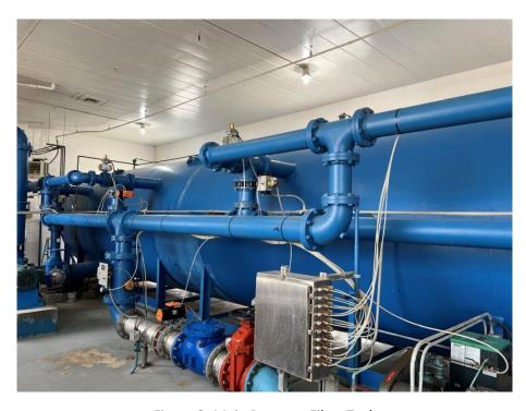
Figure 2: Main Pressure Filter Tank
